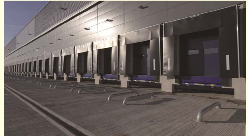
Large logistics warehouse, UK
