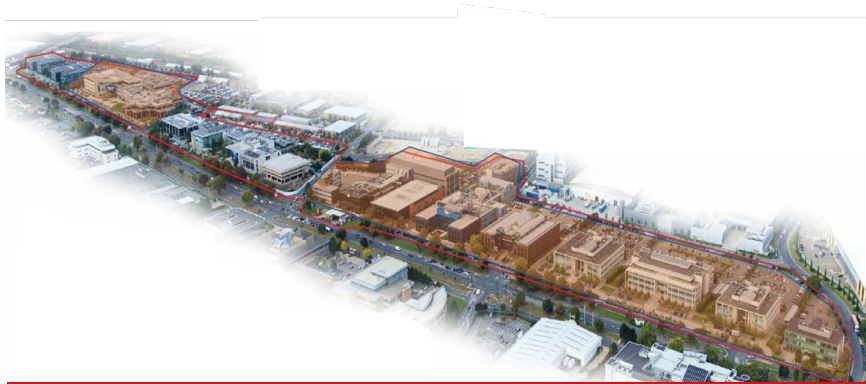
Bath Road offices
