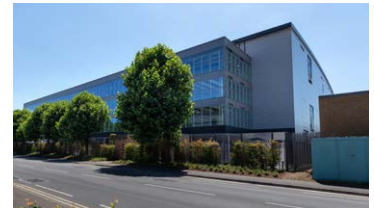
Data Centre, Slough Trading Estate, UK
