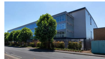
Data Centre, Slough Trading Estate, UK
