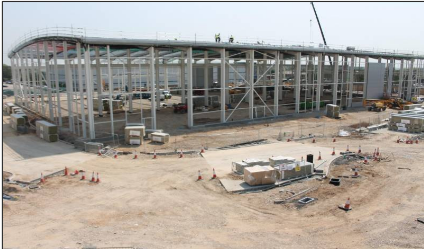
Rolls-Royce at the Portal Site, Heathrow Due to be completed December 2012
