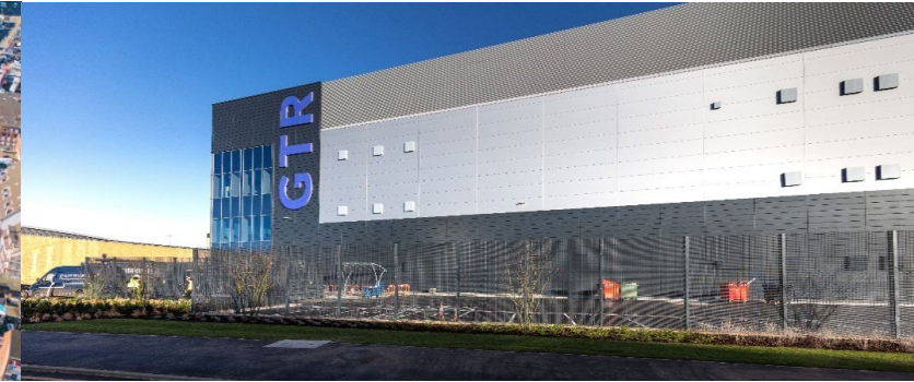
Data Centre, Slough Trading Estate
